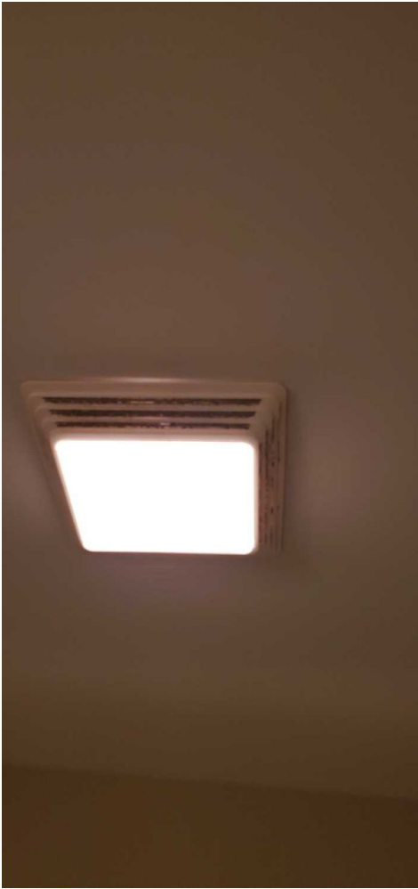
Basement West Bathroom
