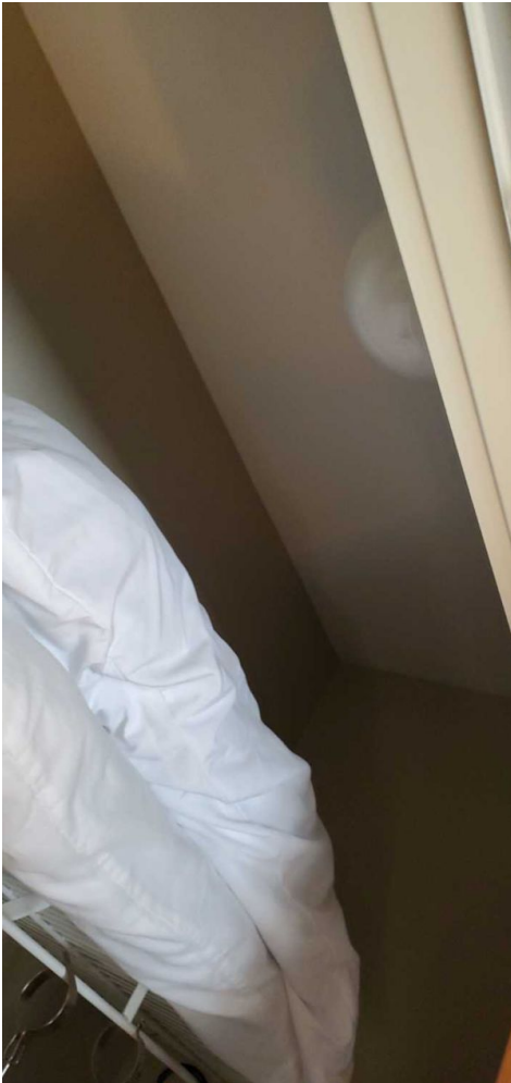
2nd Floor closet
