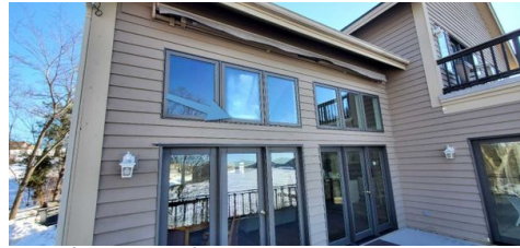
1st Floor North Living Room
