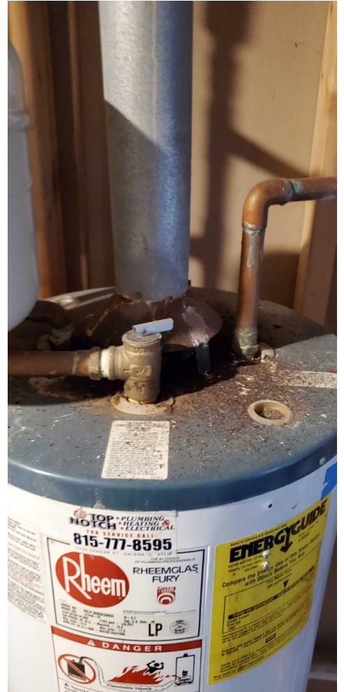
For in floor heat
