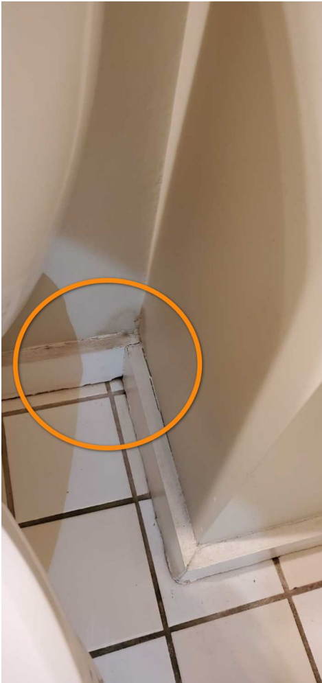
Basement West Bathroom
