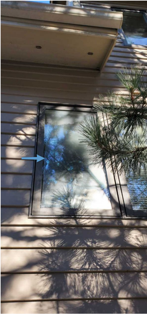
1st Floor West Bathroom
